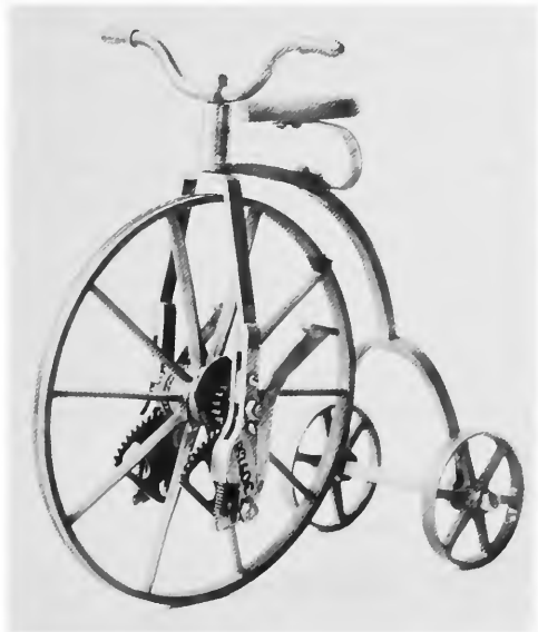
Patent Office model of the Hammelmann tricycle, 1880.
