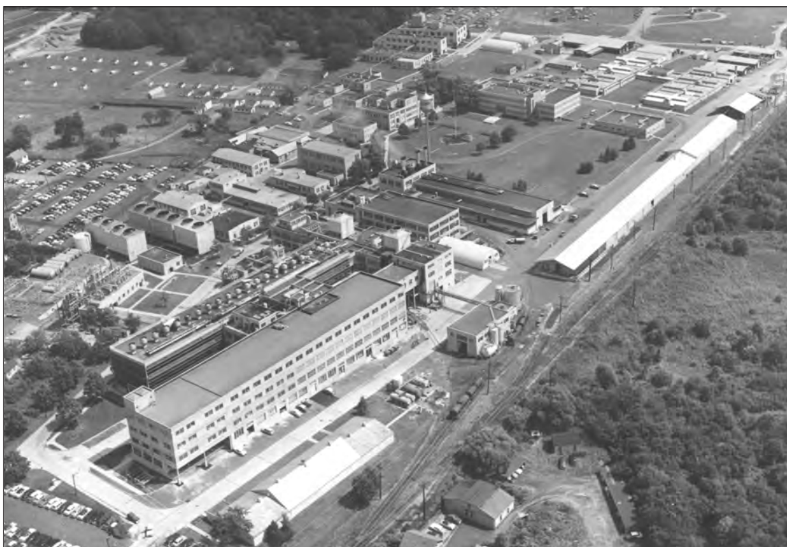
Sprawling manufacturing plants like this E. R. Squibb & Sons facility in New Brunswick, New Jersey (seen here in 1958), helped to supply mass-market pharmaceuticals after World War Two. Photograph courtesy of AIHP Drug Topics Collection.
