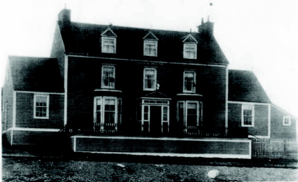
Figure 3: Undated photograph of Bridge House. Note the long veranda and wrought iron railing. Photograph courtesy of the BHTF (Mills)
