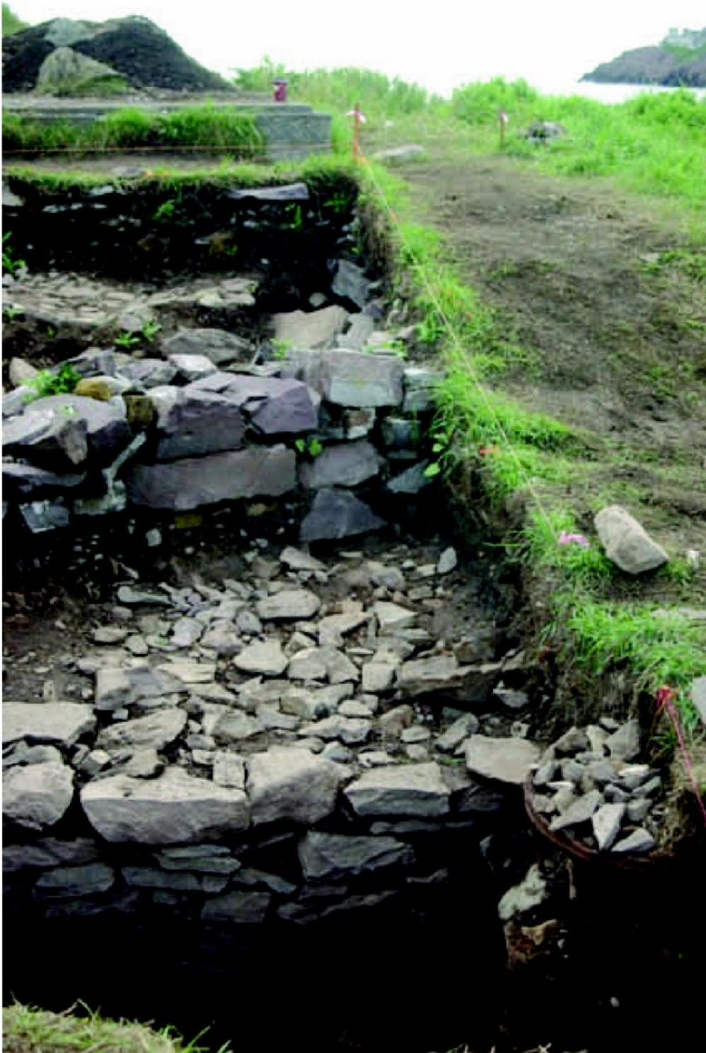
Figure 2: Artificial terrace and retaining wall (Crompton)
