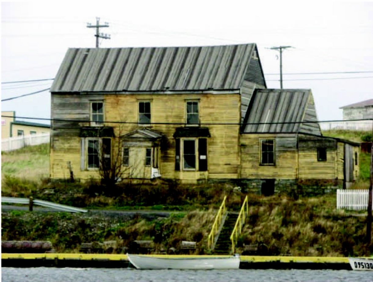
Figure 4: Bridge House in 2006 looking north. It is missing the west wing, dormers, chimneys and veranda. The pitch to the roof on the well house (right side of the house) has also changed (Mills)
