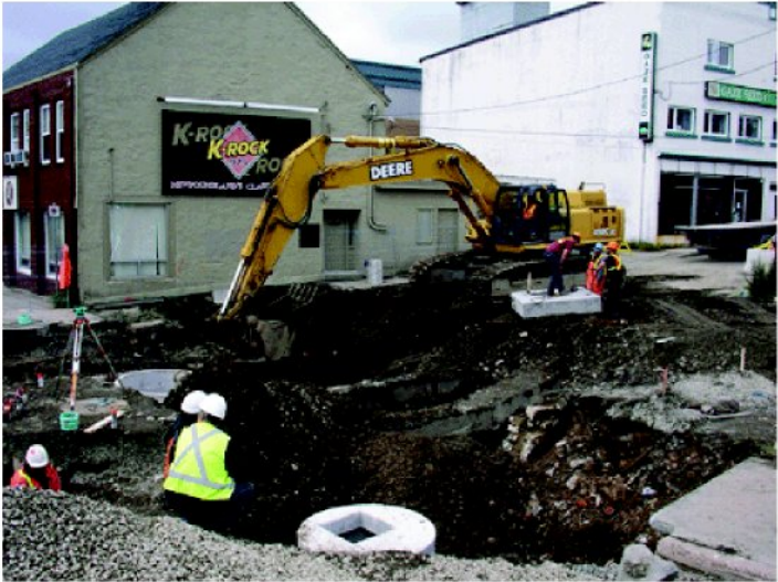
Figure 13: Phase I excavations, Buchanan Street. A mid-19 th century foundation/feature at bottom, right (CjAe-88). A 19 th century sewer can be seen at centre, left under the corner of the John Howard Society Building, which was built shortly after the 1846 Great Fire (Penney & Cuff)
