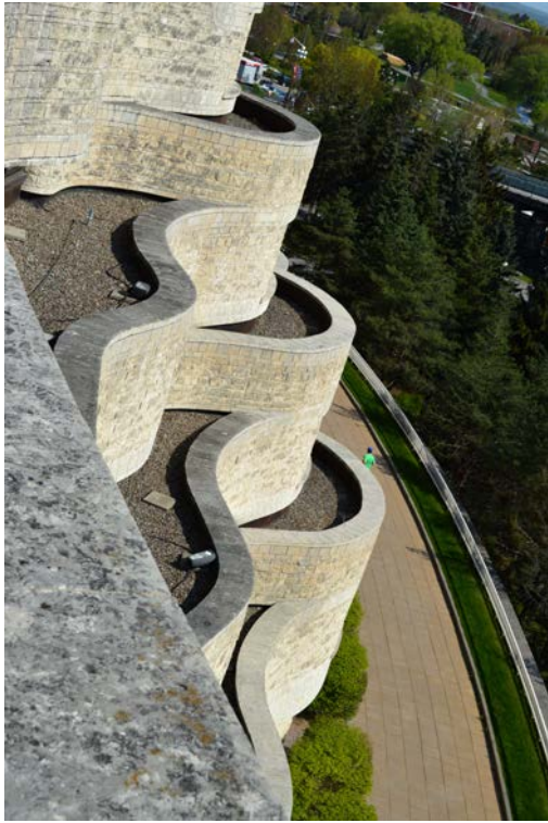
Fig. 3. CMH. Balconies exhibit dark spots on projecting stones. Biocolonization can be seen on the capstone in the foreground at left (May 17, 2017).
