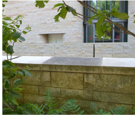
Fig. 8. NMAI, loading dock wall. Hydraulic lime parging containing zinc compounds was applied to the uncleaned pair of capstones on either side of the untreated, dark-colored "control" block at the center less than a year before this photograph was taken on June 6, 2017. The coloration of the parging could be adjusted to better match the stone. The west façade in the background was cleaned in December 2016.
