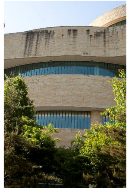
Fig. 2. NMAI, north facade. Sloping capstones contributed to severe black streaking from biocolonization below the Inouye Terrace just six years after the building opened (M. Wachowiak and E. Webb, April 22, 2010).
