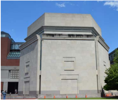
Fig. 5. U.S. National Holocaust Museum (1993). By 2000, the building's Salem Limestone had become disfigured by biocolonization. Following cleaning of the building in 2010, zinc strips installed near the edge of the roof have largely eliminated the problem on flat portions of the façade (June 2, 2017).
