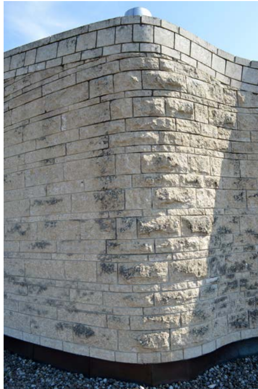
Fig. 4. CMH. Stonework on the roof of the curatorial building shows scattered biocolonization on high relief areas nearly 30 years after the building opened. Since it cannot be seen from the ground (or Parliament), it is unlikely to have ever been cleaned (May 17, 2017).
