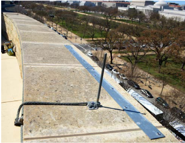
Fig. 7. NMAI, Inouye Terrace. Two years after installation, zinc strips had eliminated biocolonization on outer edges of capstones (March 31, 2014), but their effectiveness on the façade below was indeterminate because of cleaning the following month (and again in 2016). Biocolonization is also absent below the lightning rod from dissolution of copper and near joints where the stone was made water repellent by silicone caulk.
