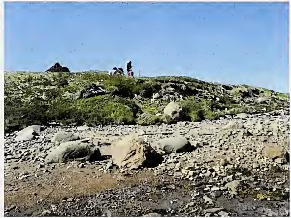
Figure 7.66 Eroding bank has destroyed the front half of House 1.
