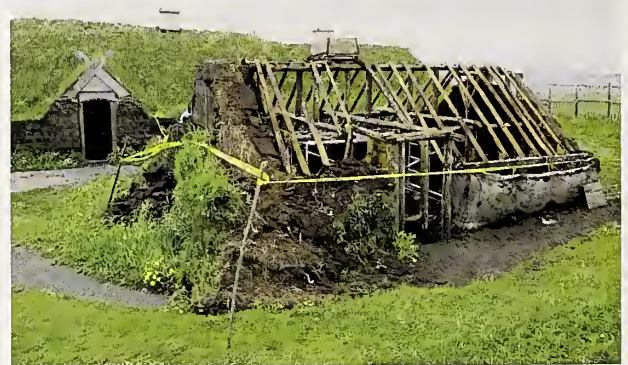
Fig 4.06: L'Anse aux Meadows Viking site out-buildings under reconstruction showing timber and sod elements.
