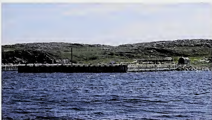
Fig 4.50: Punchbowl dock, still serviceable. View S.
