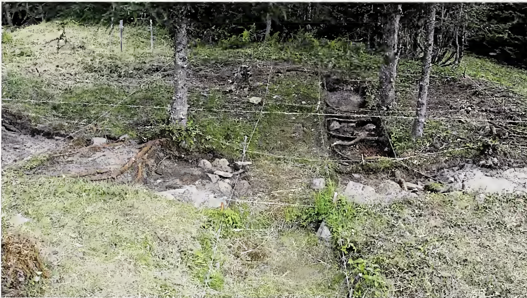
Fig 6.00: Hart Chalet (EiBh-47) House 1 looking through entry to rear wall, view north.
