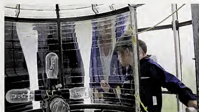
Fig 4.71: Fresnel lens at Forteau Lighthouse.
