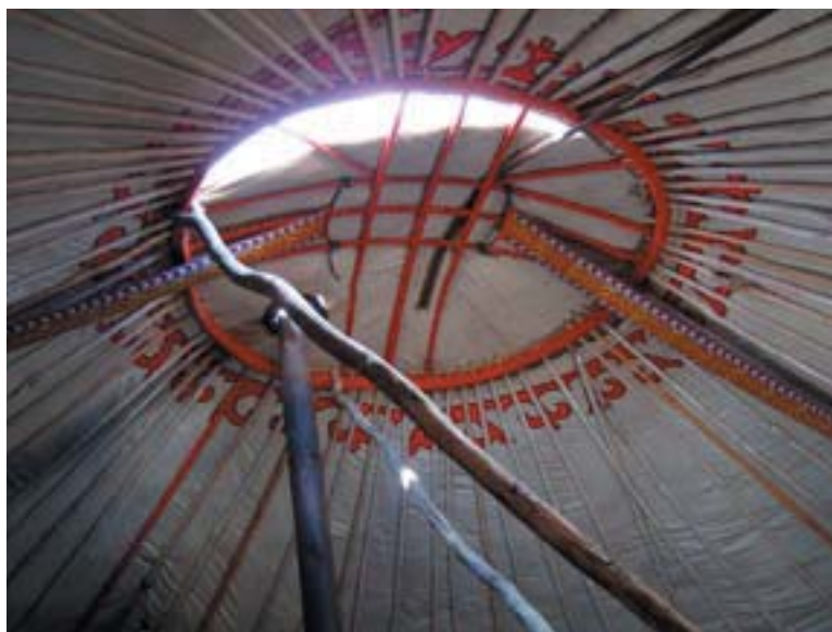
The inside of Bogdat's ger, a Kazakh-style construction variant of the Mongolian ger. (Photo: Bayarsaikhan)
