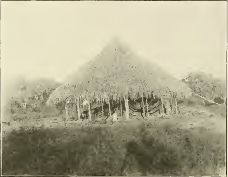
A , Circular house without side walls, Makusi, Rupununi River.
