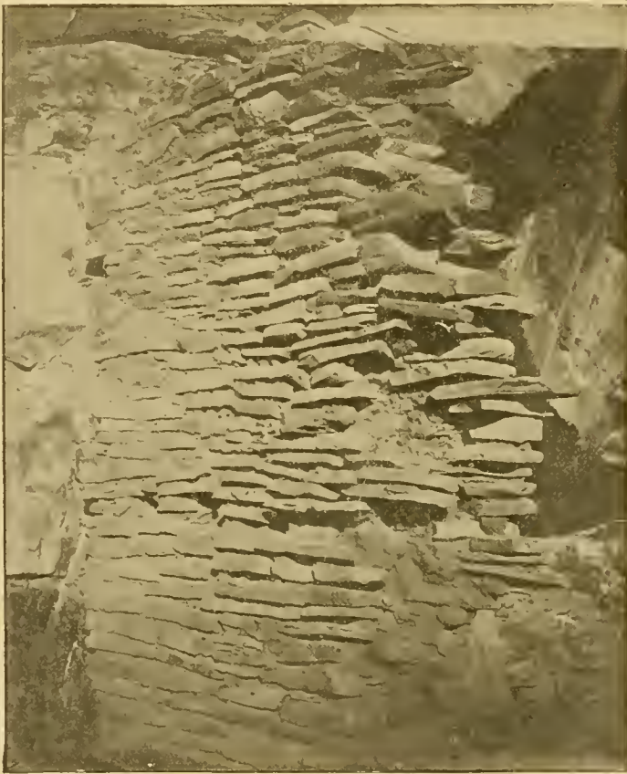
FIG. 250—Structure of wall of Honanki
