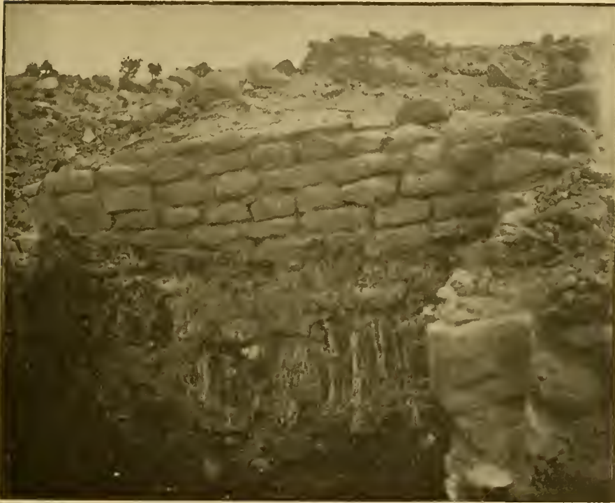
FIG. 256—Structure of house wall of Awatobi
