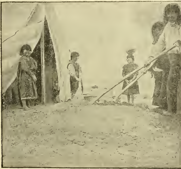
FIG. 12.—Mixing clay for plaster.
