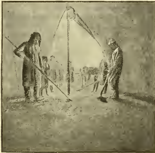
FIG. 4.—Breaking the earth under tent.
