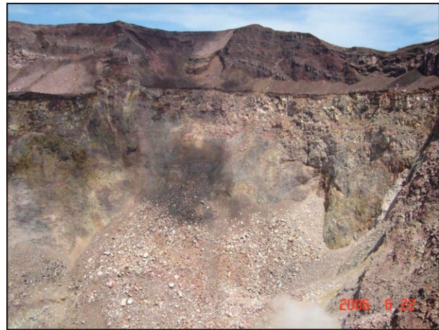
Figure 7. San Miguel's S crater wall exposes zones of altered and fractured rocks. A planar zone of structural weakness appears towards the right. Photo taken on 22 June 2006. Courtesy of SNET.
