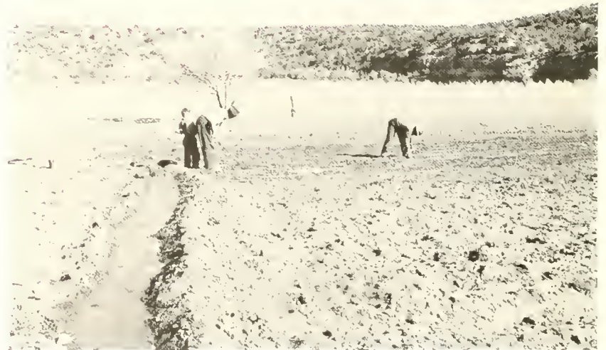
Acequias (irrigation ditches) were often dug before houses and other buildings were completed. Today, the acequia is a recognized political subdivision of the State. Photo courtesy Harvey Caplin Estate
