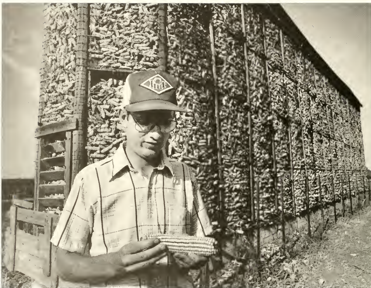
Steve inspects an ear of corn. Steve's father built this storage bin in 1972 from wire and old telephone poles. The sun and the wind dry these ears naturally, unlike the mechanical process used in closed steel bins.
