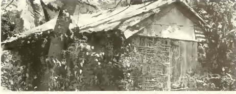
Weathered by years of hurricane seasons, an abandoned wattle and daub house still stands in St. John, its basketwork structure exposed by the elements. (Photo by Fred Nahwooksy)
