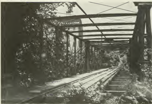
Built shortly after the Civil War, this Baltimore & Ohio Railroad bridge has been preserved as an historic engineering landmark near Savage, Maryland. An older neighbor is the former cotton duck mill behind it, which was built in 1816.
