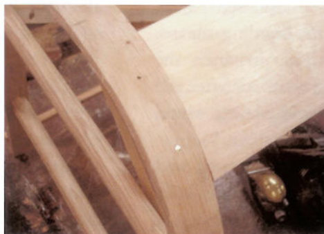
Figure 13 Large screws protruded through the face of the presentation surface and were simply filed flush.
