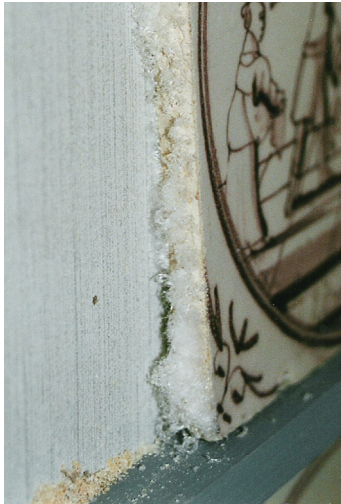
Figure 4. Thick layers of fluffy efflorescences growing on Dutch tin-glazed tile (inv. 3922). Left of the tile there is a heap of debris, fallen off another tile
