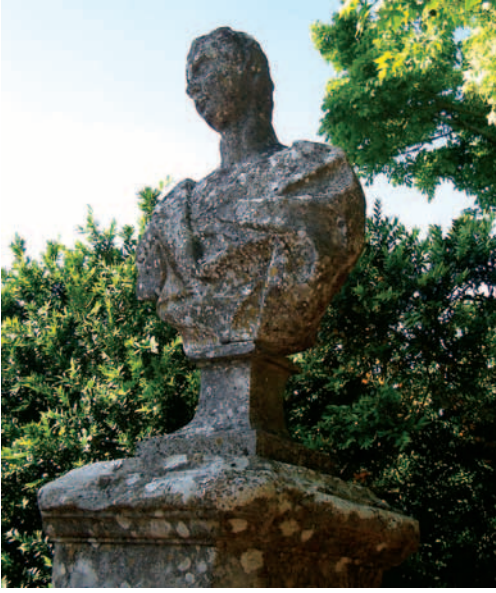
Fig. 2, a, b. Aspects of the heavy biocolonisation in the stone sculptures.
