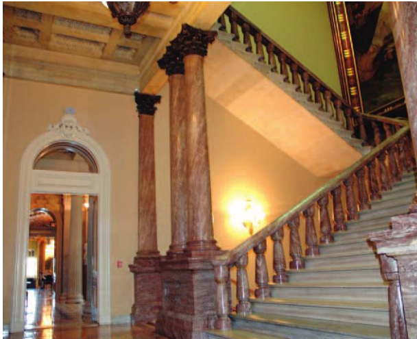
Fig. 7. Cornelius and Baker, Senate staircase capitals, US Capitol, 1855. Zinc and brass. (Photo, Carol Grissom.)
