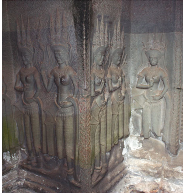
Fig. 4.20 Salts partially originating from bat guano at Angkor Wat (Cambodia)
