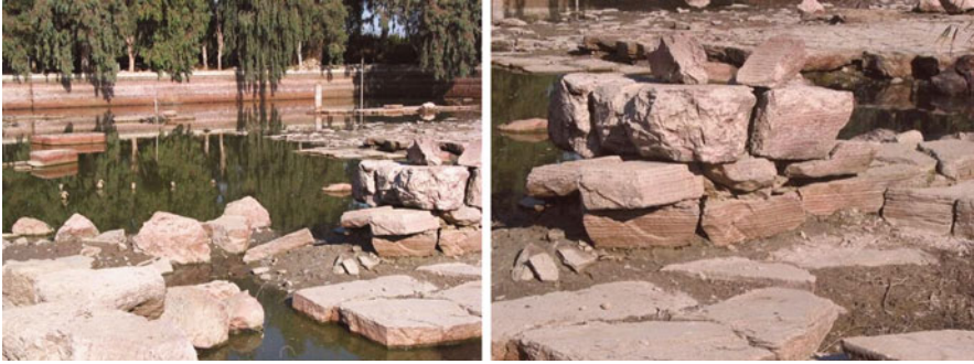
Fig. 4.30 Ephesus, Turkey: the rosy stain on white calcareous limestone is caused by bacteria forming blooms in the brackish water of the pond overlaying the subterranean parts of the Artemision
