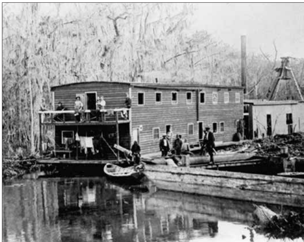
The Bowie Lumber Co. operated this quarterboat and dredge in Louisiana in the early 20th century. Southern lumber companies built canals that enabled them to harvest trees in cypress swamps via pullboats. (Photographs courtesy of the Forest History Society Photo Collection)
