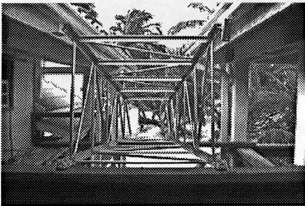
Fig. 6: Tower shown in horizontal servicing position. At this point of the installation, the lower half of the tower is attached to the platform as an exercise designed to verify that sufficient clearance is available between the roof and tower during rotation.
