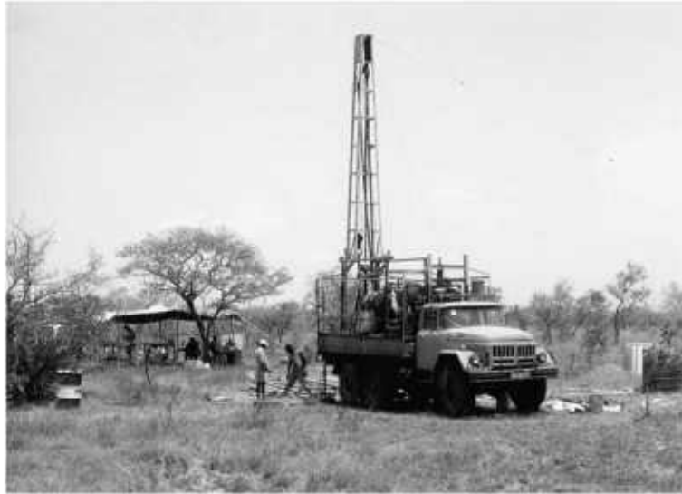
Fig. 2. Photograph of drilling operations at TDP Site 3, showing the truck-mounted rig and mobile field laboratory (background).
