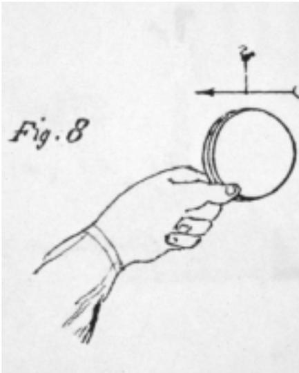
Figure 2. Demonstration of the deflection of a magnetic needle by the “thermoelectromagnetic” action of disks of two different metals held between the fingers. From Yelin 1823c.
