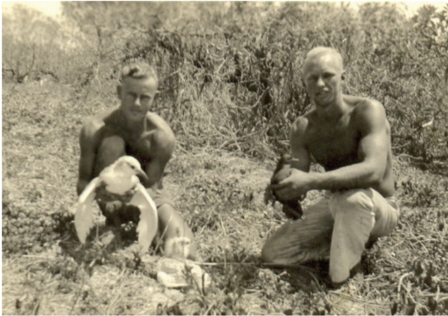
Figure 5. Construction workers with a bo'sn bird and a dark shearwater, maybe Christmas? Peale Island-1936 (photo courtesy of C. Nickerson).
