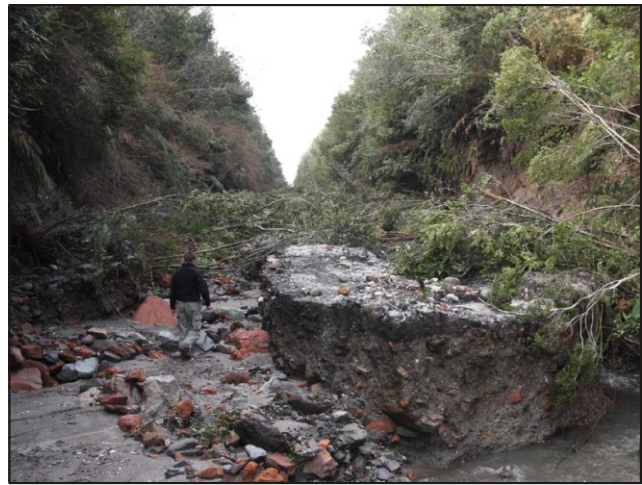
Figure 3. Drainages redirected by Chaitén's eruption caused erosion of this road to the volcano's N. Courtesy of Richard Roscoe, PhotoVolcanica.com.
