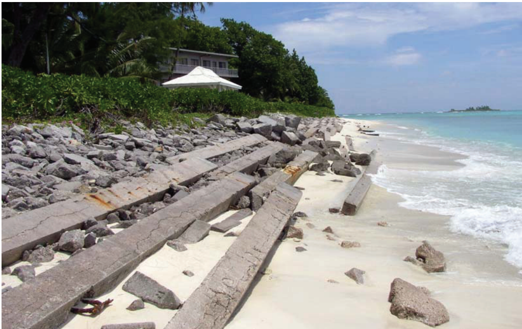
Figure 4. Northern tip of western Diego Garcia showing concrete armouring against erosion. The reef flat at this site is over 100 m wide. View looking North.
