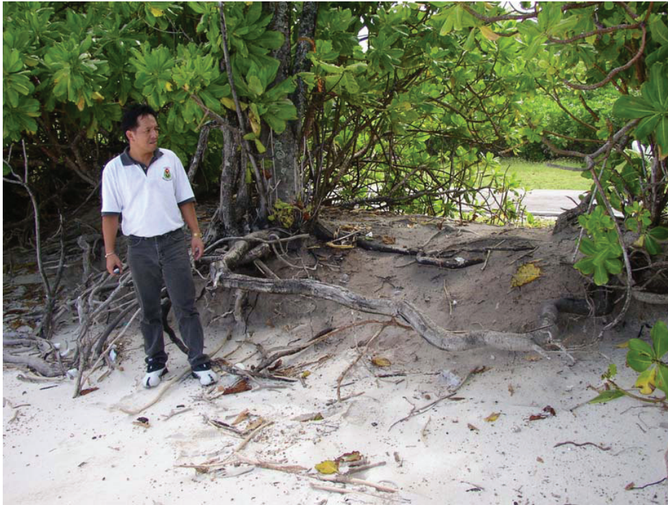
Figure 5. Erosion of the seaward side of the western arm of Diego Garcia. The observer is standing on the high tide level, the thin rim behind him is now all that stops inundation of the road at this point.
