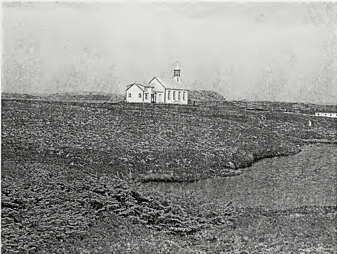
Fig. 5.49: Providence church, to northeast
