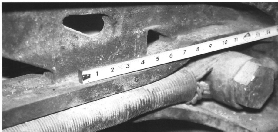
Fig. 1. Continuous wire-wrapped wire cable at one bearing end of Gries-Gendell (Severson) girder in Smithsonian collection. All photographs by the authors.
