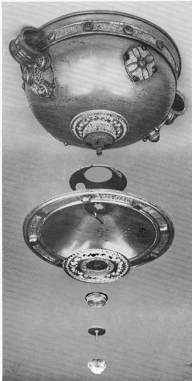
25. An exploded view to show how the components of the chalice were reassembled temporarily in 1962.
