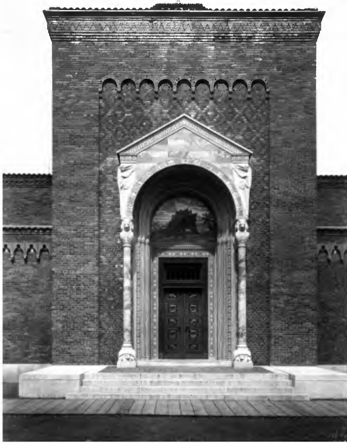
FIG. 1. Photograph of Reptile Building at National Zoological Park shortly after completion in 1931. Credit: National Zoological Park Photo Archives.
