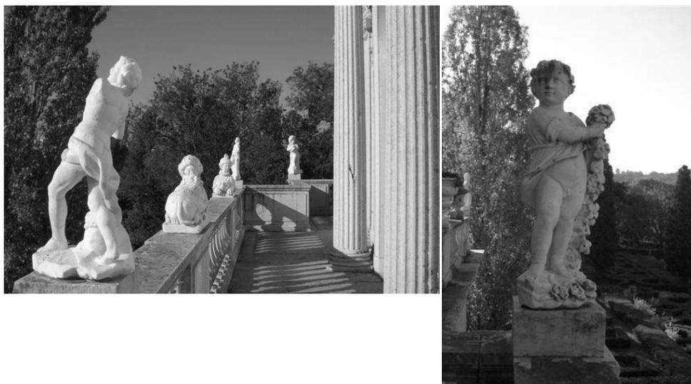
**Figure 5:** Statues on the terrace balustrade treated with an aqueous emulsion of an oligomeric siloxane after cleaning in 1999. On the left, one of these statues shows development of bio-colonization on the more exposed head. Photos 2007.
