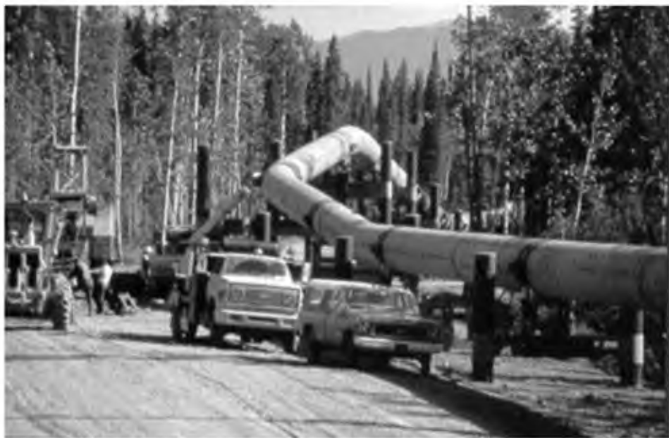
To avoid damaging areas of unstable permafrost, nearly 420 miles of the 800-mile-long Trans-Alaska Pipeline were built above ground. (Photo courtesy of the Alyeska Pipeline Service Co.)
