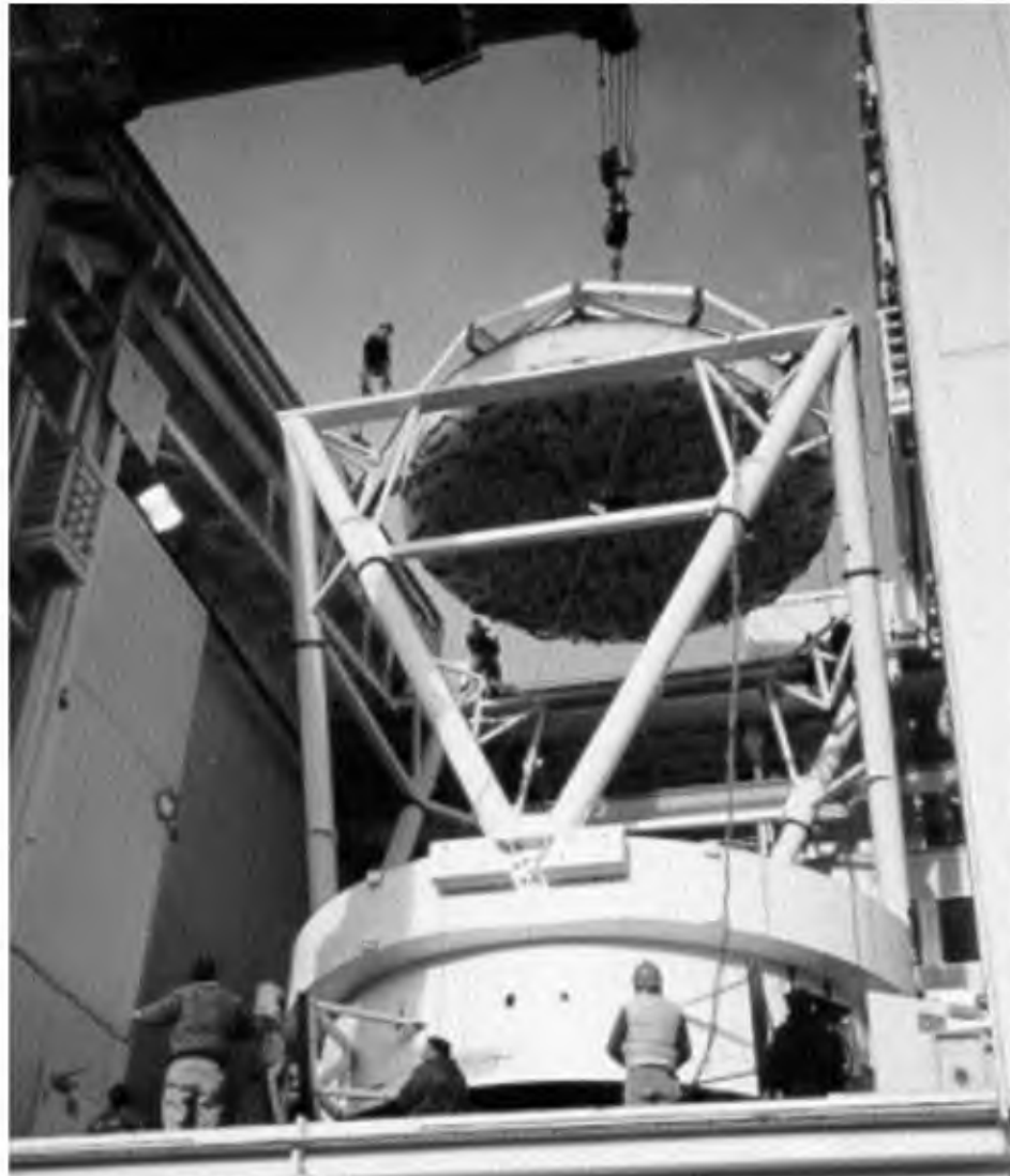
In a remarkable feat of engineering achievement and high-altitude logistics, staff from the Smithsonian Astrophysical Observatory guide the replacement mirror through the narrow confines of the telescope struts and into the support structure and cell below. (James Cornell photo)
