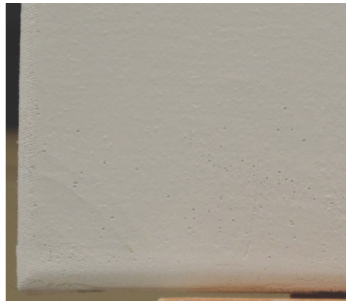
Figure 13. Sample 5. After 14 RH sets corner BC had 2 cracks plus 1 faint crack
