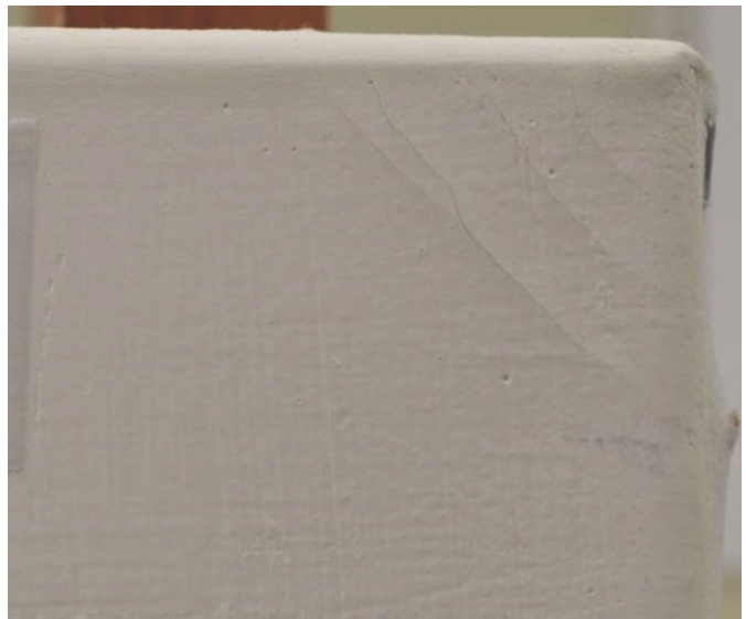
Figure 10. Sample 3. After 14 RH sets, corner AD had 3 cracks
