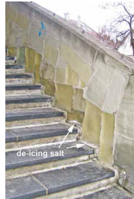
Figure 1: Lausanne (canton de Vaud, CH), Pierre Viret stairs (20.01.2010). Deicing salts are spread lavishly on the practically non-porous gneiss, and the salt and melted snow mixture accumulates at the base of the porous molasse-sandstone bridge wall that promptly powders and disaggregates.
