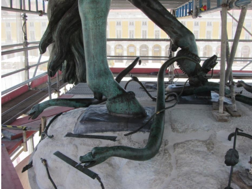
Figure 8. Aspect of the top of the plinth showing the fractures sealed and the visible bronze clamps treated.
