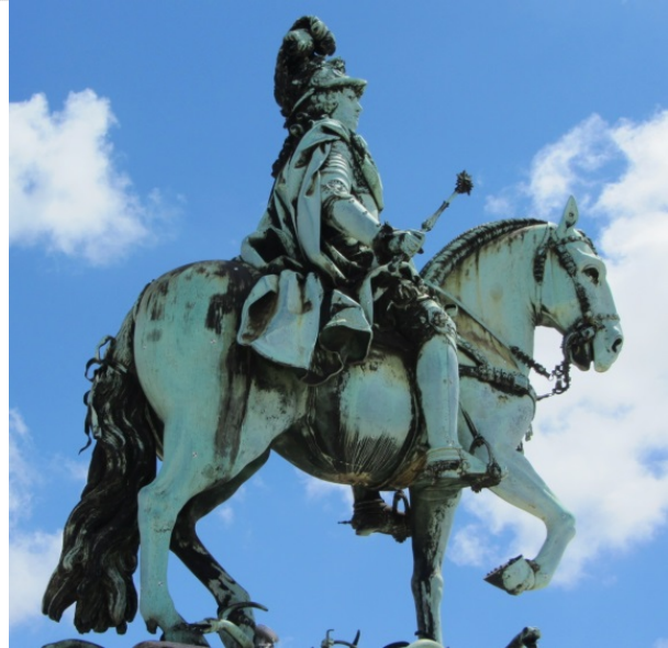
Figure 1. D. José I statue in Lisbon. East view (left) shows the prevalence of dark patinas, while in the west side (right), more exposed to the marine winds and rains, green patinas prevail.
