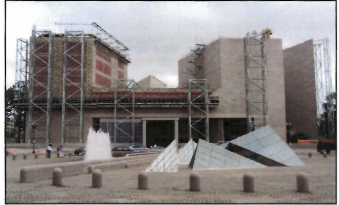
Figure 35. National Gallery of Art East Building during removal of 10-cm-thick blocks of Tennessee marble in 2012, subsequently replaced using new anchors.
