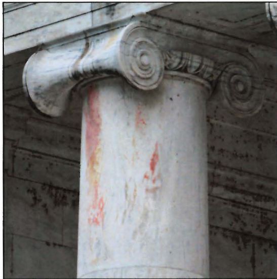
Figure 19. Detail of a Shelburne Marble ionic capital, Jefferson Memorial. Horizontal cracks visible in the volute have resulted in falling stone from some columns. Biological staining can be seen on the wall behind.
