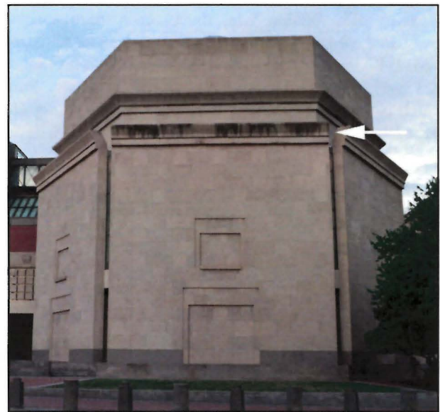
Figure 20. U.S. Holocaust Memorial Museum, Salem Limestone. Zinc strips installed in 2010 have reduced black biocolonization except in the area indicated by the arrow, where they were not installed.
