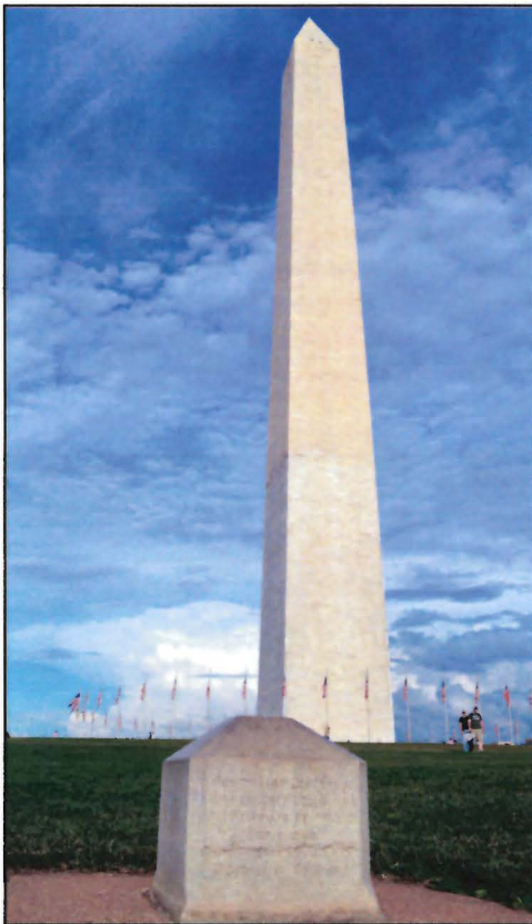
Figure 14. Washington Monument, showing Texas marble on the bottom third and Cockeysville marble on the upper two thirds. The Jefferson stone is in the foreground. Compare with the 1851 view in Figure 2.
