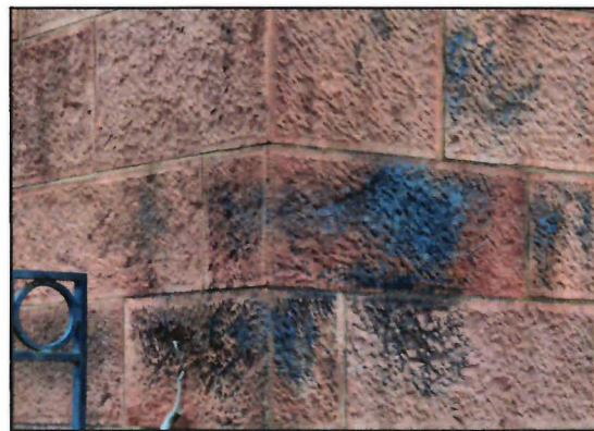
Figure 22. Dark blue–black patches on the Seneca sandstone , southwest corner of the Smithsonian Castle, on which X-ray fluorescence spectrometry found elevated manganese. The block with the darkest patch measures 71 cm in width.
