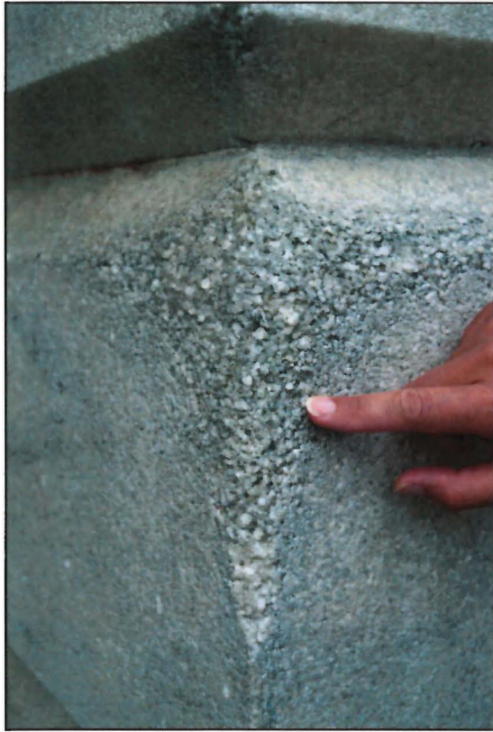
Figure 8. Texas marble corner, Patent Office Building. Erosion at grain boundaries shows the coarse texture of the stone.
