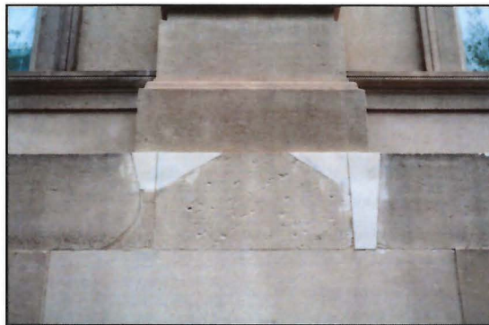
Figure 12. U.S. General Post Office/Hotel Monaco, Westchester marble . Corroding iron cramps between blocks below corners of the pilaster resulted in the crack at left and dutchmen (stone infill). Pockmarks in the center block (81 cm wide) are from weathering out of tremolite.
