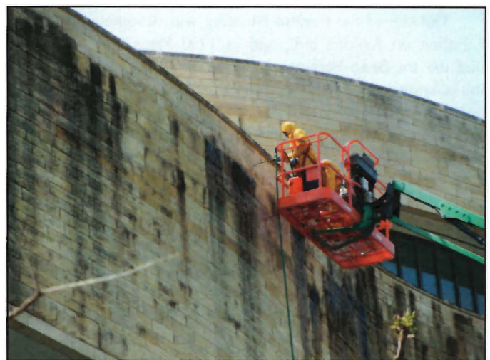
Figure 26. Cleaning biocolonization with a biocide from the Kasota stone on the National Museum of the American Indian in April 2011.
