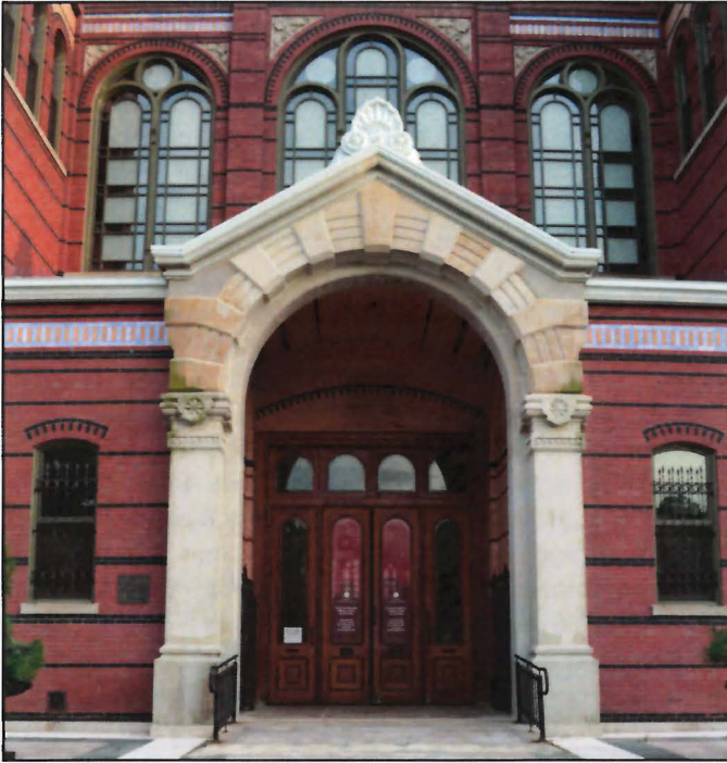
Figure 23. North entrance to the Arts and Industries Building, Euclid bluestone . Iron staining on the archway is typical of the stone. Bases for the shafts were replaced with Buena Vista Sandstone around 2009.
