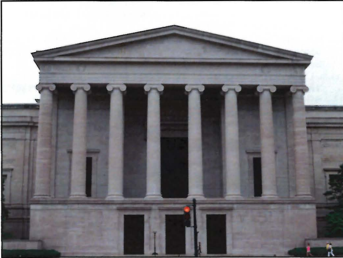
Figure 34. National Gallery of Art West Building, Tennessee marble . Note stronger banding on outermost columns.
