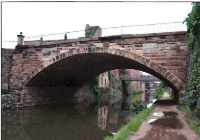
Figure 5. Wisconsin Avenue Bridge over the C&O Canal, Georgetown, Aquia Creek sandstone .
