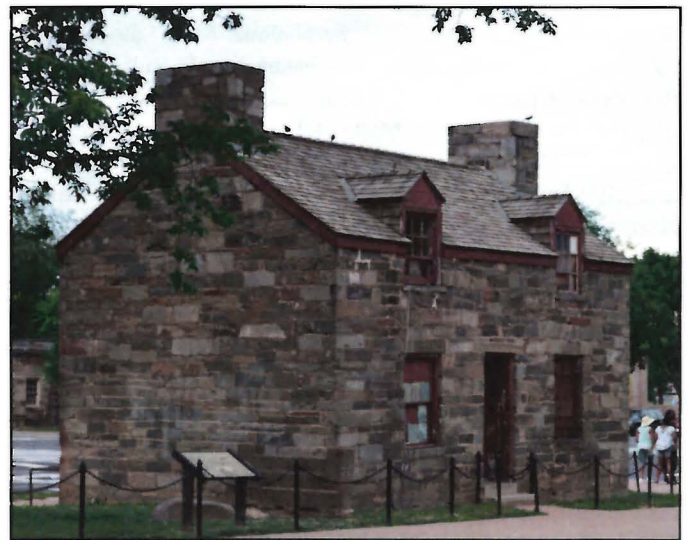
Figure 18. Lockkeeper's house, Potomac bluestone .
