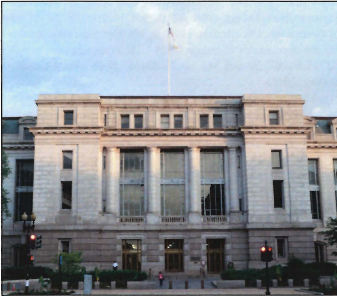
Figure 13. National Museum of Natural History. Ground floor is Milford Granite; next two floors, Bethel Granite; and top floor, Mount Airy Granite.
