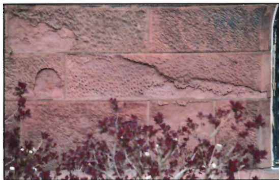
Figure 21. Detail of Seneca sandstone , west façade of the Smithsonian Castle. Central block (206 cm wide) shows retooled surfaces after multiple delamination.
