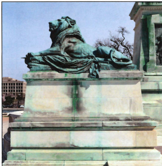
Figure 30. Copper runoff from the Grant Memorial's bronze Lion has left disfiguring green and purple stains on the Vermont marble base.
