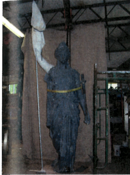
Fig. 5. Liberty from Goldsboro, NC, with replacement arm and flag model. These were then molded, re-created in zinc sheets using the repoussé method and soldered to the original before gilding. Conservation Solutions, Inc.
