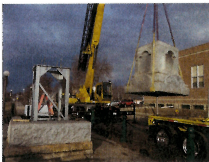
Fig. 10. Monument in New Ulm, MN, during re-assembly on supporting armature. Conservation Solutions, Inc.
