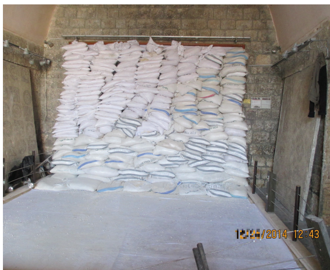
Figure 5 (below). Reinforced and stabilized mosaics at the Ma'arra Museum, December 2014. Photograph source anonymous for protection.
