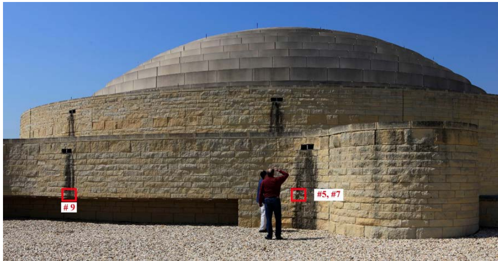
Figure 2. Left, view of the east face of the 5 th floor terrace showing locations of samples #5, #7, and #9 from darkened areas below two scuppers, which drain water from the small terrace above and, in turn, the main roof terrace with the dome (April 2010).
