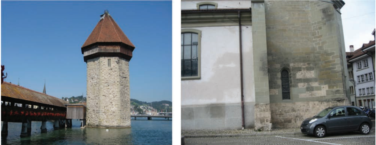
Figure 5: Left: Tower at the Kapellbrücke on the Reuss river, built with Molasse sandstone some 700 years ago. Even though the tower has its foundations sunk into the bed of the river, no rising damp is observed. Right: Detail of the Basilique Notre Dame, Fribourg, where damp areas are found up to about 4–5 m high. The Basilica was built by the former infilled moat of the Castle; nearby there had been a cemetery, and later, on market days, animals would be standing there contributing to enrich the soil with salts while deicing salts are used in winter.
