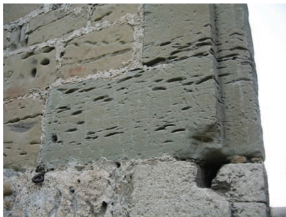
Figure 10: Molasse sandstone in the Fribourg city wall. The Burdigalien formation often contains inclusions of very fine-grained marl (a calcareous mudstone) with fine pores that tend to weather out first.
