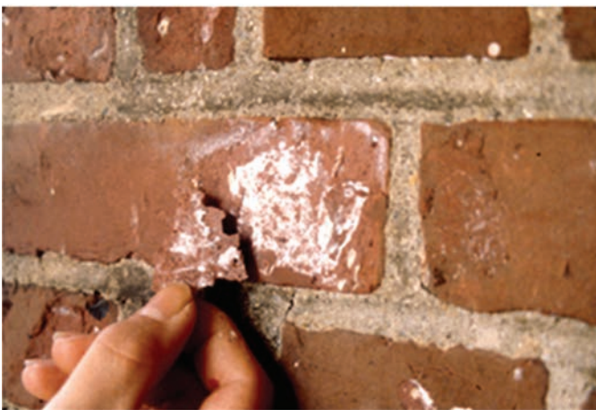
Figure 2: Left: Sodium sulfate crystallizing at the subsurface in brick masonry causing the detachment of the flake that is being held showing the salt present also on its underside. Right: Portal at the Manhattan College in New York City, where this occurred. Figure 3 provides further information about this damage.
