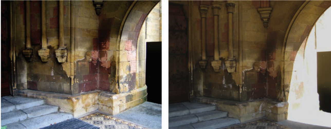
Figure 11: Western porch of the Collegiale of Neuchâtel (Switzerland). Left shows a detail of the wall on a relative humid day in October 2009; Right, the same detail on a relative dry day in April 2010. Salt efflorescence from a mixture of sodium sulfate, gypsum and sodium chloride is clearly visible on both figures. The wall on the left, at higher RH, shows damp halos around the efflorescence from the deliquescence of all salts; on the right, at lower RH, the sodium chloride deliquesces by taking up the water from the sodium sulfate decahydrate thus showing slightly less efflorescence. (Images and information by Bénédicte Rousset).
