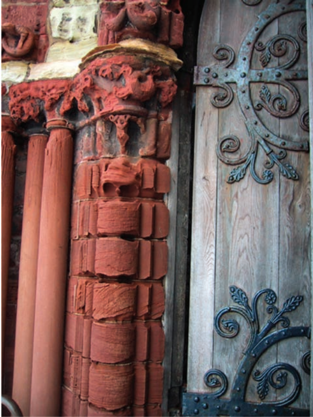
Figure 1: Typical weathering patterns caused by salts (granular disintegration and alveolization) on sandstone at the portal of St. Magnus Cathedral, Kirkwall, Orkneys.
