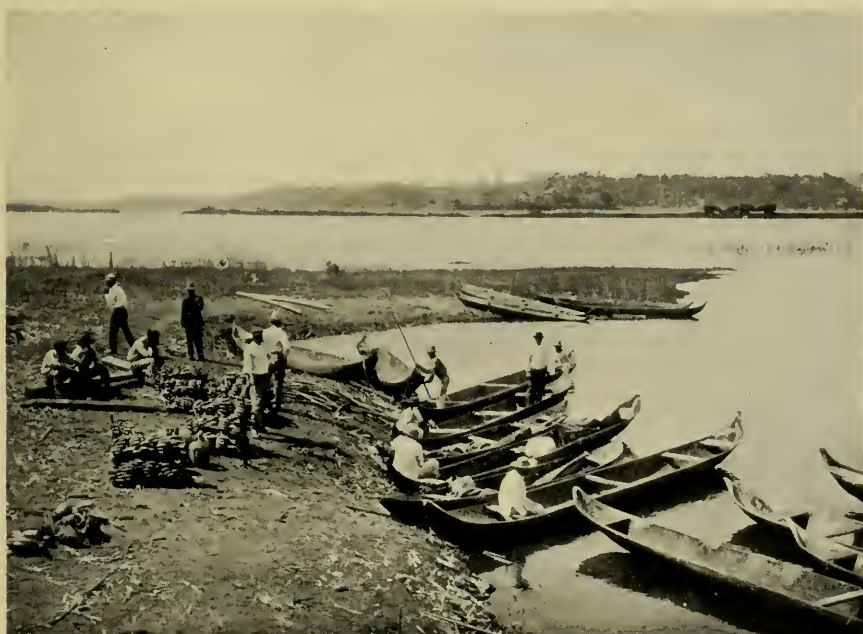
FIG. 2.—Gatun Lake with water rising. New canoe landing near Gatun; old line of Panama Railroad in distance, April 30, 1911.
