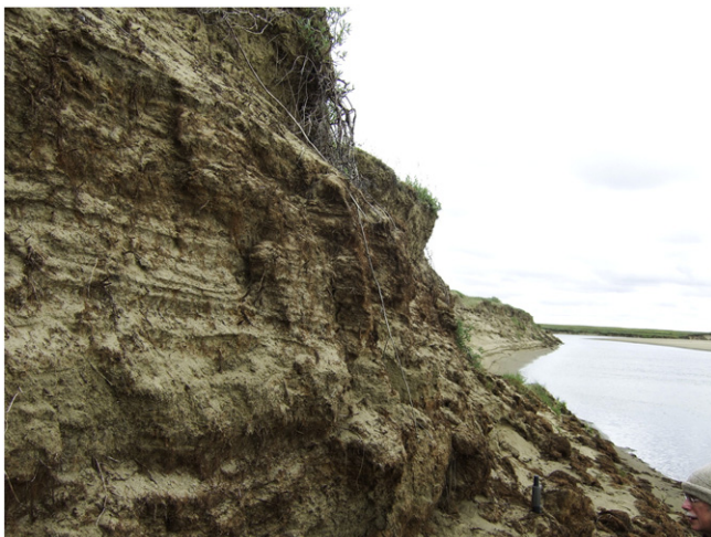
Fig. 14. Dense network of fine plant roots extending from the shrubs beyond the crest of the bank. See Fig. 12 for location.
