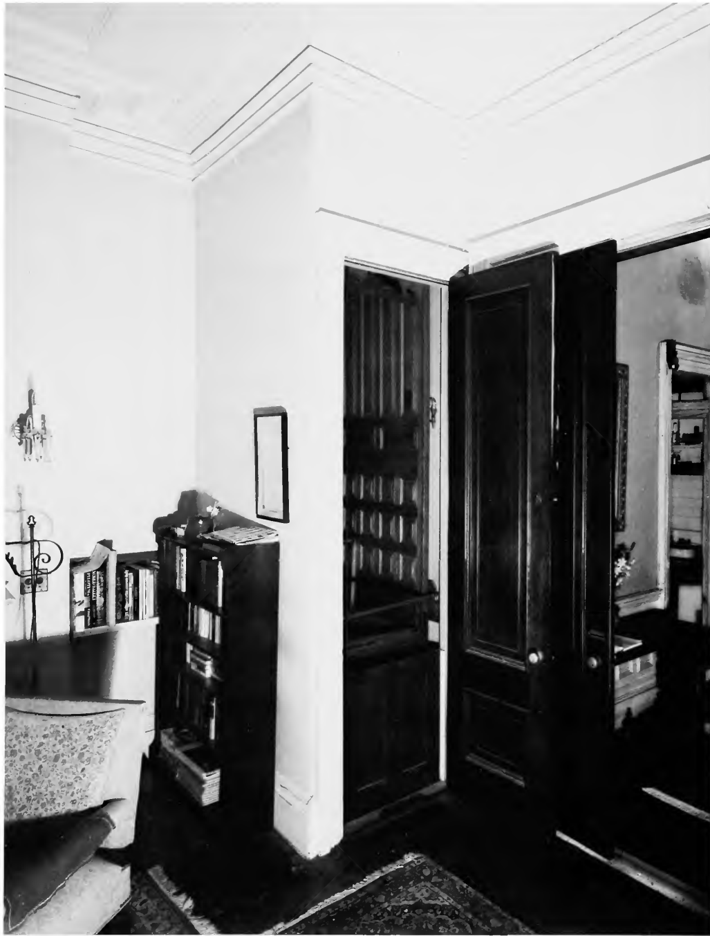
FIGURE 10.—The Wheeler elevator in its final resting place just above the second-floor level, where it reposed, unmoving, from 1942 until its ultimate removal in February of 1985, having settled there as a result of the “jam.” The small panel was fitted to prevent objects (and people) from falling down the shaft from the space beneath the car. The stacked closets on the house’s first three floors seem to have been planned almost with a future elevator shaft in mind. As a result of this feature, minimal architectural modification was required when the elevator was installed some 36 years later. The original closet doors served readily as the elevator shaft doors. Against the right shaft-door jamb, mid-height of the car, is seen the gas cock to which was attached the flexible rubber hose that supplied gas for the car’s ceiling light in the original installation. The hose and light fixture were removed, presumably when the house was wired sometime after the elevator was installed. (Jet Lowe photograph for the Historic American Engineering Record, 1985.)
