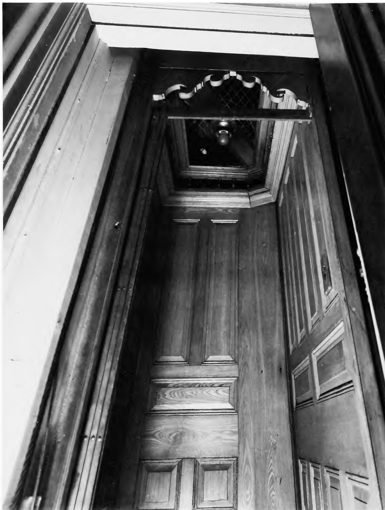
FIGURE 11.—The car interior. All is original except the ceiling light, its switch, and the folding car gate which probably was added at the insistence of the city's elevator inspector. (Jet Lowe.)
