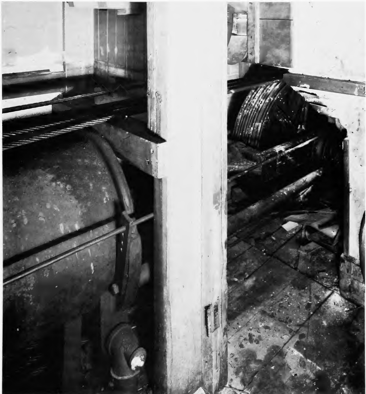
FIGURE 14.—The traveling sheaves and their inner guide rail, tucked neatly beneath the bottom run of the basement stairs. (Jet Lowe.)
