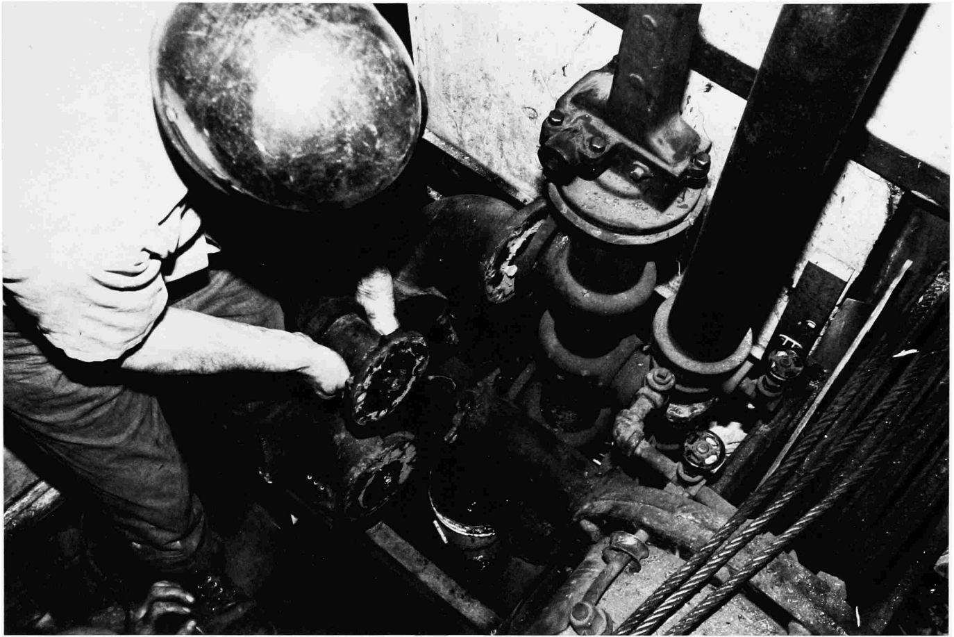
FIGURE 16.—Manitou Machine Works crew dismantling and removing the operating valve, February 1985.
