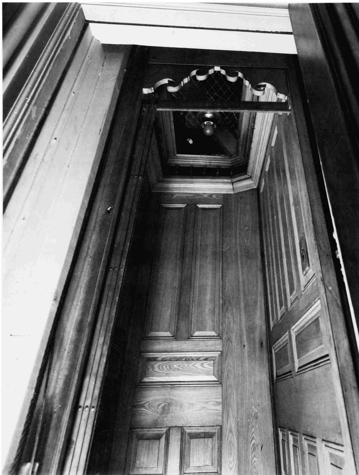
FIGURE 11.—The car interior. All is original except the ceiling light, its switch, and the folding car gate which probably was added at the insistence of the city's elevator inspector. (Jet Lowe.)
