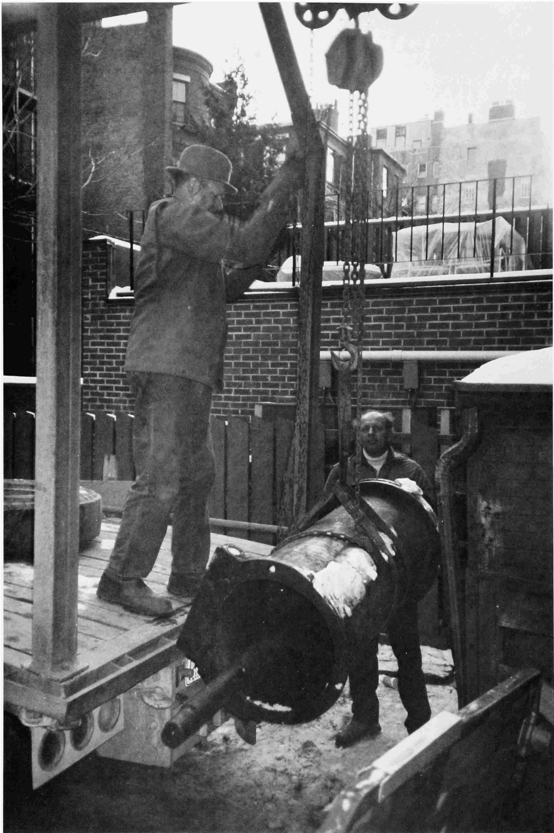
FIGURE 17.—The power cylinder with its piston and piston rod being loaded. The fatal, final “jam” in the system lies here, for the piston defied all attempts to move it within the cylinder during the removal process.
