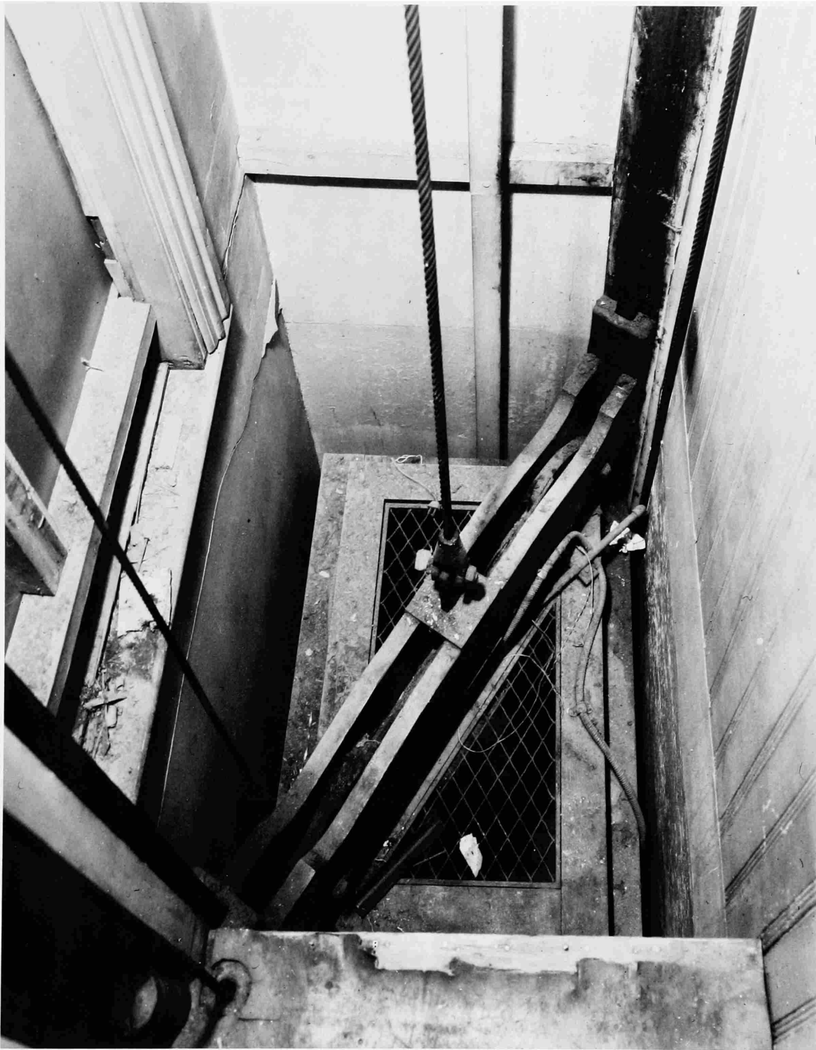
FIGURE 12.—Looking down on the car from the third-floor level, showing the diagonally set guide rails; the attachment of the single hoisting rope to the Otis-type broken-rope safety within the hoisting beam; the part of the hoisting rope running between the basement and the overhead hoisting sheave (to the right of the rear guide rail); and the two parts of the operating-rope loop (at left). On the car roof are seen the armored cable for the electric light and adjacent to it the gas pipe for the original light, left in place when the modification was made. (Jet Lowe.)
