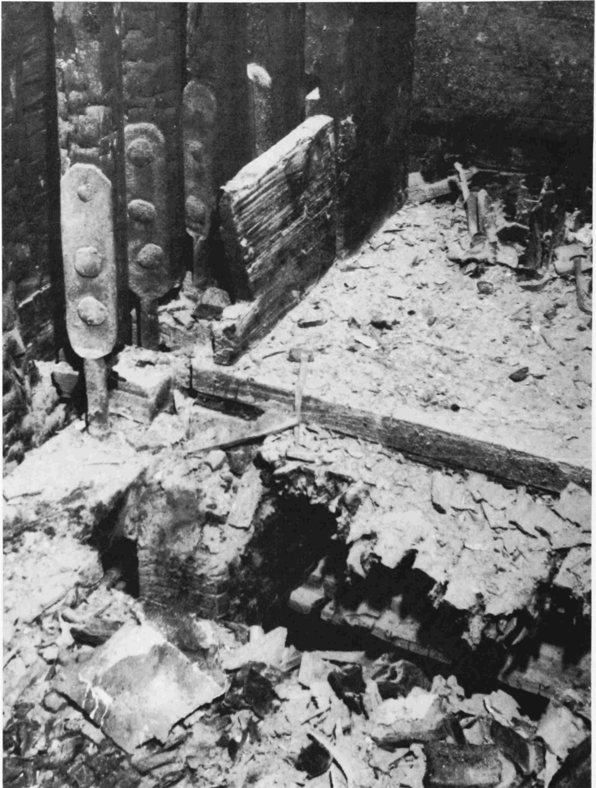
FIGURE 10.—Epistle organ, Cadereta, before the restoration of 1975–1978 shows extensive fire damage.
