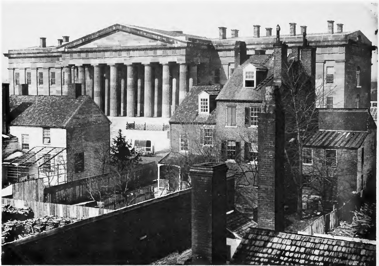
Figure 25. —THE UNITED STATES PATENT OFFICE, CA. 1846. This classic marble structure, begun in 1836 following the destruction of the original Patent Office by fire, was completed in 1840. In addition to housing several government bureaus including the Patent Office, it became the repository of four museum collections, including major exhibits from the Wilkes and Perry expeditions, the varied acquisitions of the National Institute for the Promotion of Science, and miscellaneous donations from individuals. Its exhibits included Franklin's cane and printing press; Washington's sword, uniform, field chest, and campaign tent; and the memorabilia of James Smithson—national treasures subsequently to be incorporated in the collection of the Smithsonian Institution.
