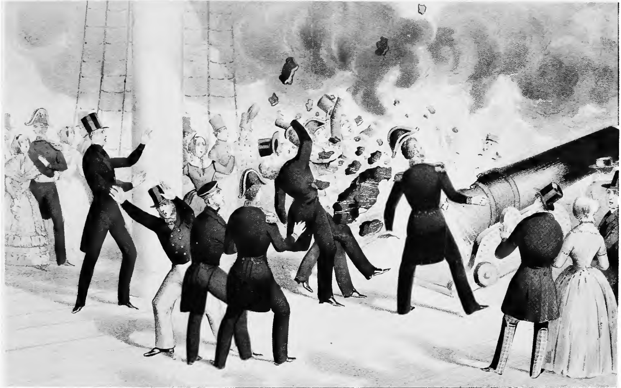
Figure 33. —THE Princeton DISASTER, 28 FEBRUARY 1844. President John Tyler, who had witnessed the first demonstration of Colt's Submarine Battery at Washington in 1842, observed the first two test firings of Captain Robert F. Stockton's flawed 12-inch "Peacemaker" on board the Princeton before the fatal salvo was fired.
