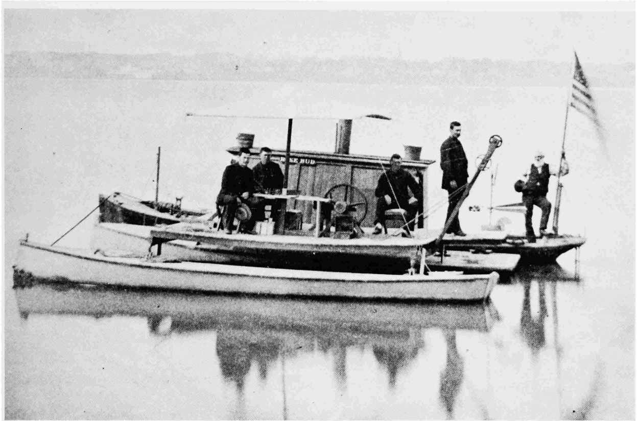
FIGURE 84.—The catamaran used by W. G. Price in 1882 for measuring the flow of the Ohio River at Paducah, Kentucky. Note current meter next to Price, second from right at stern of boat. (Courtesy of W. G. Price, Jr.)
